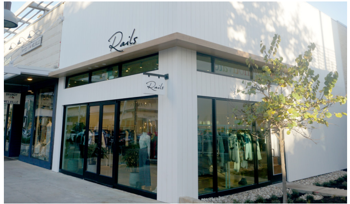
RAILS Austin, TX Superintendent: Jack Tatum Project Manager: Nick Pavletic
